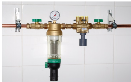
RPZ Option F and wall fixing brackets – providing rear clearance as required by the Water Regulations
